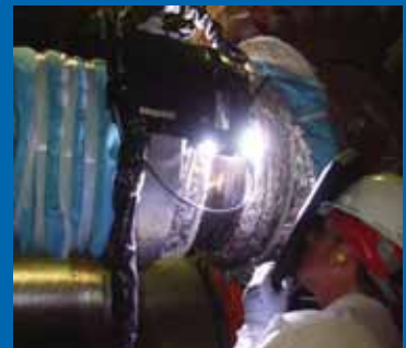
Above: A critical weld in a nuclear power plant being performed by Tri Tool Thermal Services™ with Tri Tool's new DualARC™ dual-process TIG-MIG orbital weld head and OrbitMaster™ Digital Programmable Welding Arc Controller.
