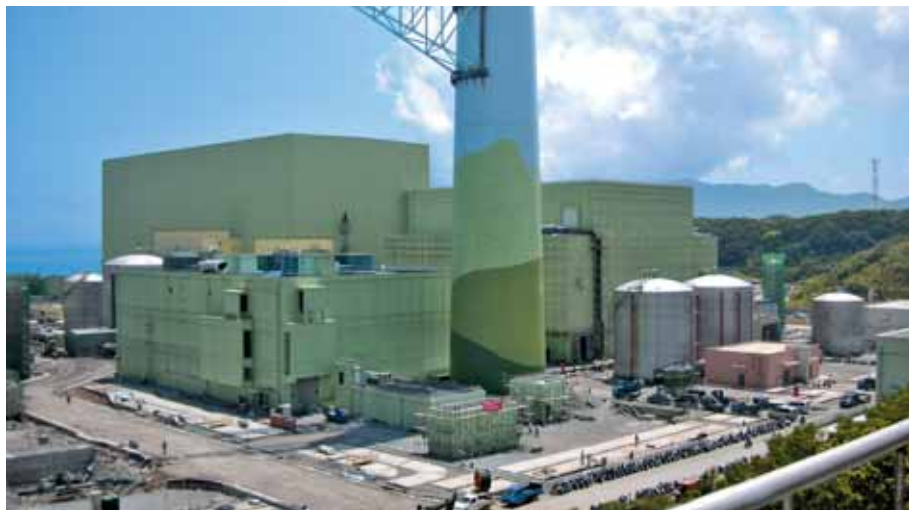
The Lungmen facility features Advanced Boiling Water Reactor technology, and when both units are completed, will be rated at 2,700 megawatts.
